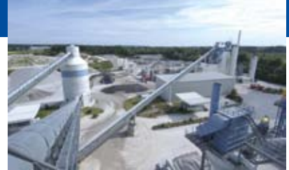
Fully automatic feeding of concrete and asphalt mixing plants
