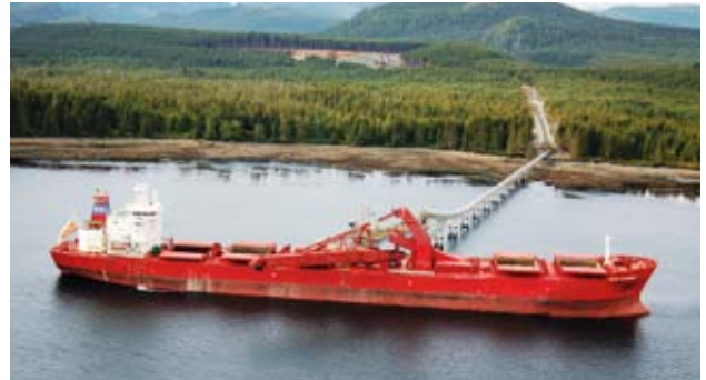
ORCA ship loading facility, Canada
